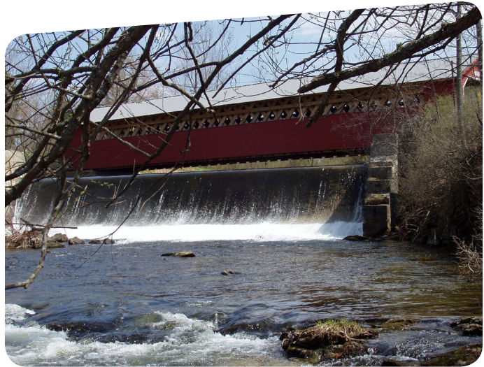
"Vermont Tissue" property – Bennington, Walloomsac River. BCRC provided over $100,000 in assessment and clean up funds. Following completion of extensive site assessments and remediation work, the site is now generating hydroelectric energy. The balance of the former mill building is being occupied by a new craft distillery.
